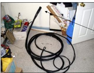
All coax's were run through the attic and fished down the wall in the new shack.
